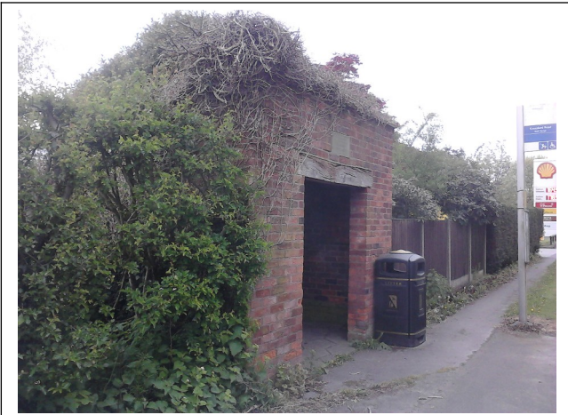
Bus passenger shelter before maintenance work – vegetation growing onto shelter roof, weeds at the entrance to the shelter and debris within the shelter.
