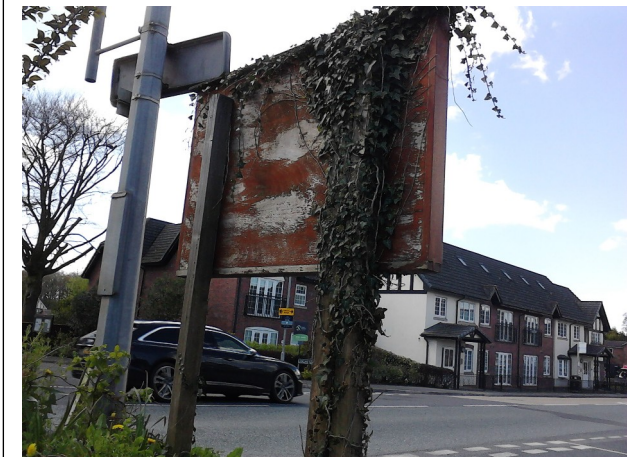
Notice board before maintenance work – deteriorating wood stain, ivy growing on supporting posts.
