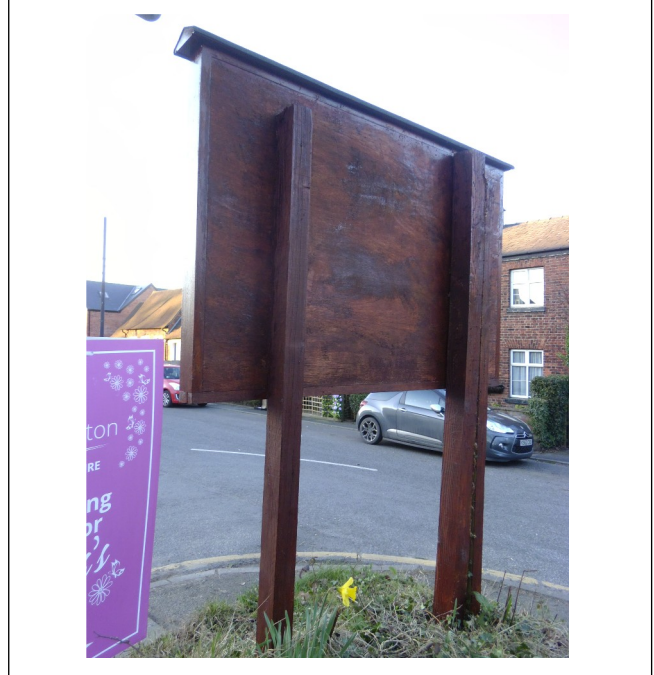
⇒ Notice board following maintenance work – woodwork re-stained, ivy removed from supporting posts.
