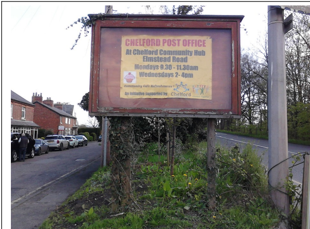
Notice board before maintenance work – deteriorating wood stain, ivy growing on supporting posts.
