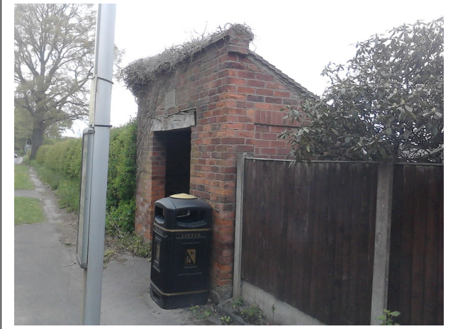
Bus passenger shelter before maintenance work – vegetation growing onto shelter roof, weeds at the entrance to the shelter and debris within the shelter.
