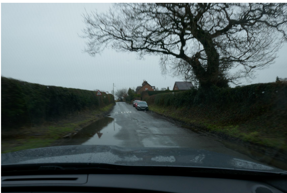
PEPPER STREET LOOKING SOUTH – NOTE ROAD NARROWS SIGNAGE
